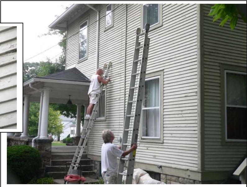
Preparation Included Hand and Machine Scraping and Abrading, Power-washing and the Application of XIM's Peel Bond
