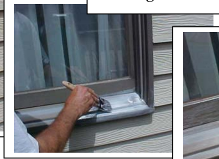
Priming Window Sills and Frames
