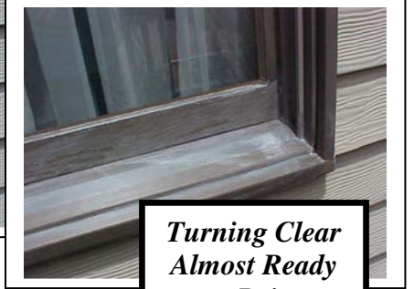
Priming Window Sills and Frames
