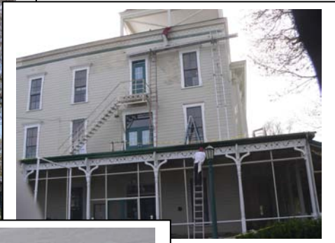
During the Job
